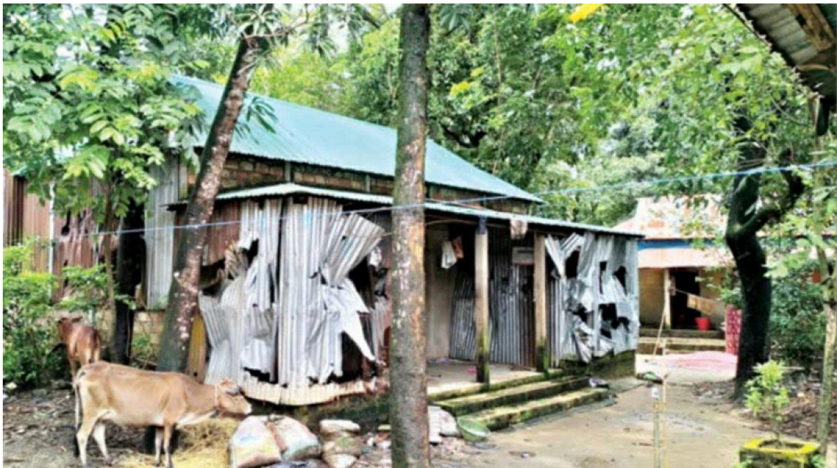
Photo: Hundreds of people attacked and vandalized Hindu community homes. They looted furniture, water pumps, tanks, and other belongings.
